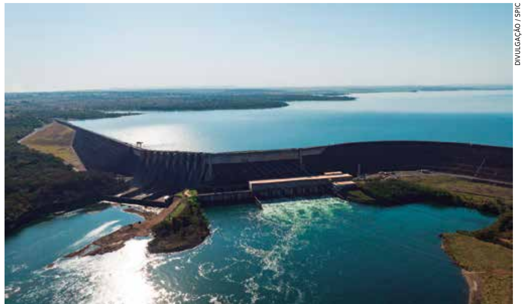
USINA HIDRELÉTRICA SÃO SIMÃO (DIVISA DE MG E GO) | SÃO SIMÃO HYDROELECTRIC POWER PLANT (BORDER BETWEEN MG AND GO)
